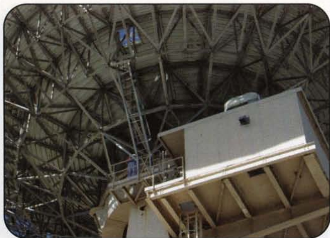
The underside of the Jamesburg Earth Station Dish in Cachagua Valley, California (about 20 miles southeast of Monterey), a 10-story tall, 97-foot diameter dish. This view shows the ladder to the access hatch and top surface of the dish. The operations room is to the right. (Photo by KB8VAO)
