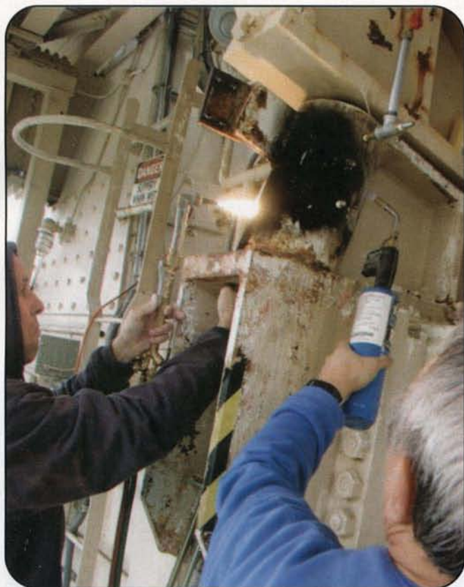
Bryan Klofas, KF6ZEO, and Brian Yee, W6BY, using heat to loosen the stow pin. (Photo by WB6DCE)
