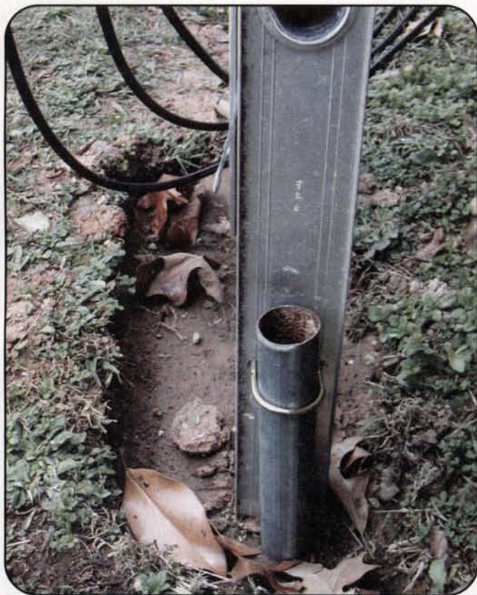
Photo 4. Base-pipe attachment scheme.
